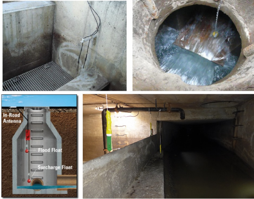
Figure 1: Different types of low-cost sensors for sewer system monitoring. From top left clockwise: i) Electrical switch at overflow crest (Rasmussen et al., 2008), ii) Motion detector at leaping weir (Siemers et al., 2011), iii) Motion detector iv) Flood float (www.123mc.com)
