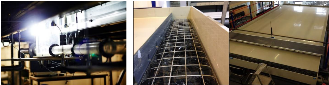
Figure 2. Below ground system consisting of a pipe connected to a manhole (left). Urban surface to which the manhole is connected (right) and the inlet tank (medium) with baffle materials.
