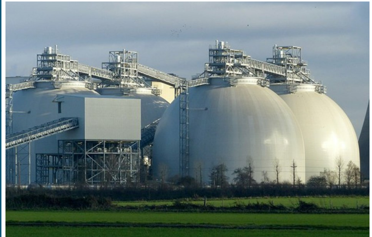
Biomass silos at Drax power plant in North Yorkshire. Drax are hoping to be one of the first large-scale BECCS projects in the world.
