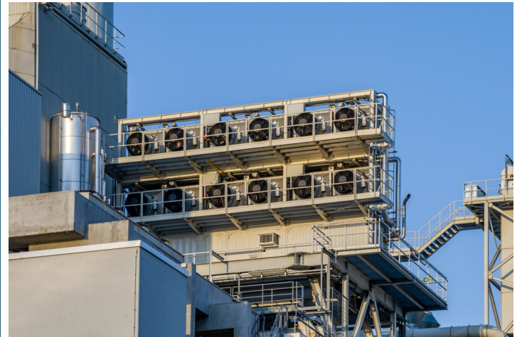
The ClimeWorks plant in Switzerland, one of the world's first full-scale Direct Air Capture projects. Image: Getty
