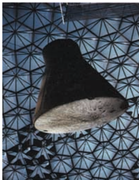
Fig. 10. Photograph (by Robin Whyman) of the inside of the EXPO ’67 dome in Montreal. One of the pentagons necessary for closure is clearly visible in the middle section, as is the way in which the strut lengths have been adjusted to achieve a smooth round shape.
