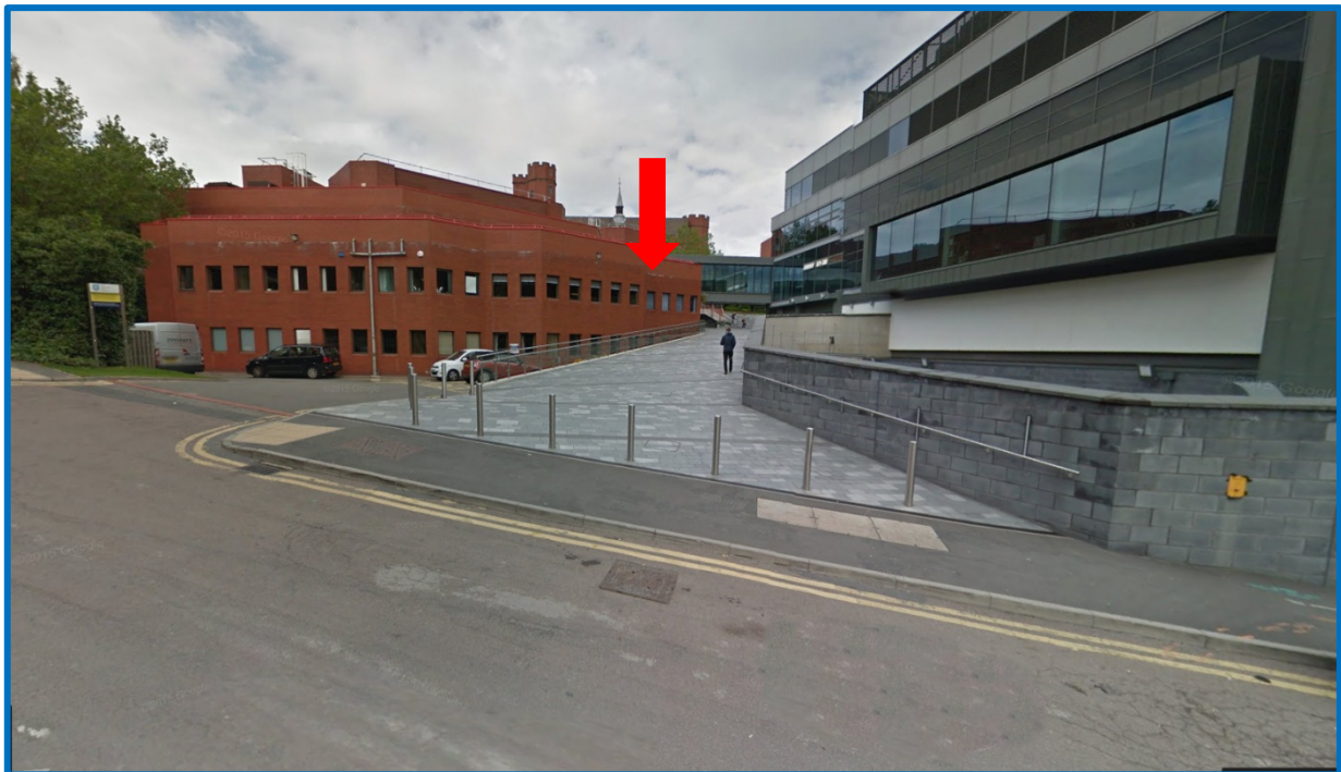
Octagon Centre from Durham Road (looking toward Firth Court)
