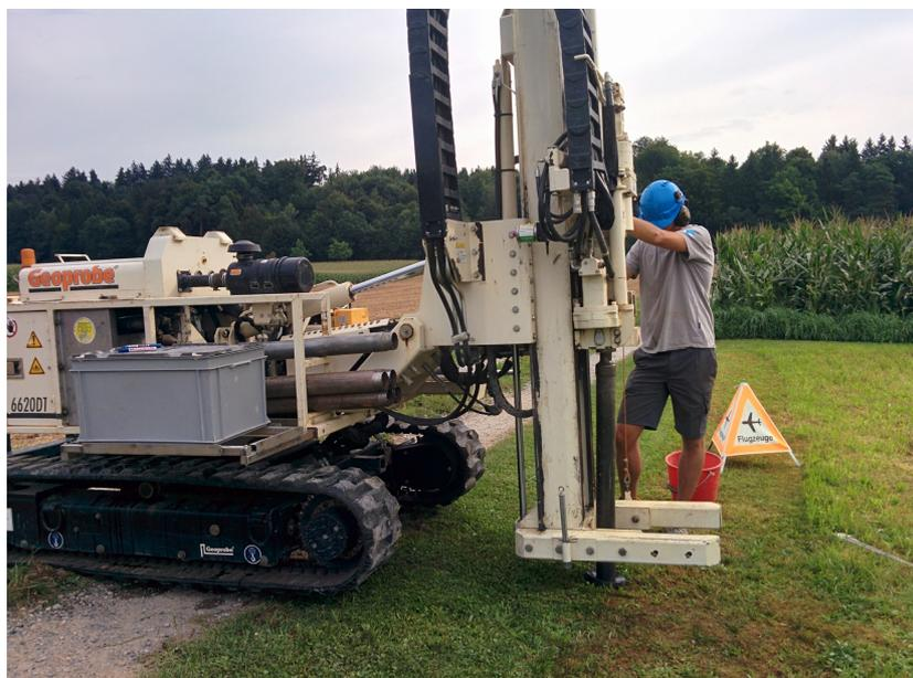
*Figure 2: Typical illustration of monitoring well installation*
