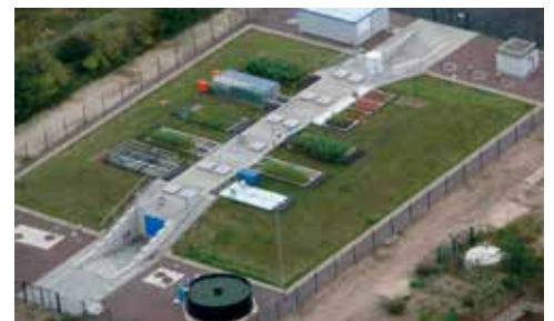
Fig. 2: The pilot scale plant in Leuna (courtesy of M. Kaestner)
