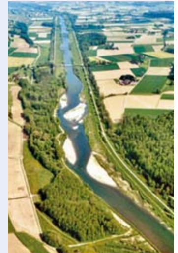
Figure 7. River Thur after restoration
