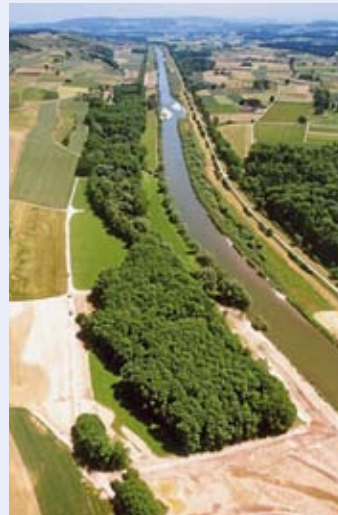
Figure 6. River Thur before restoration
