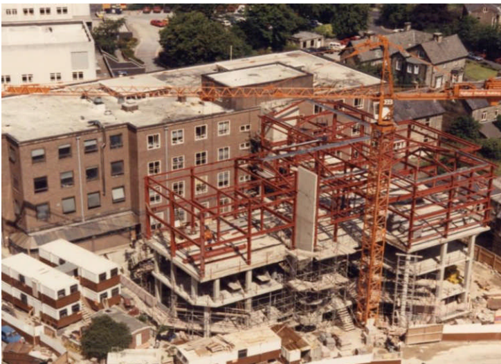
School under construction 1991
